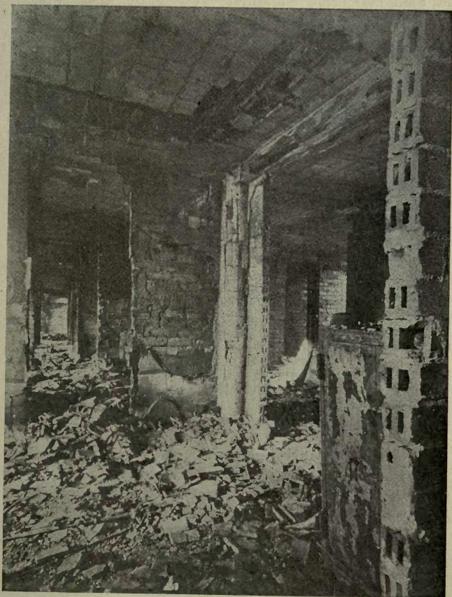
FIG. 96.—Granite Building Fire. View on 8th Floor.
